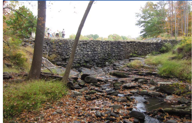
Schoonmaker Lake Dam, Blooming Grove, NY
