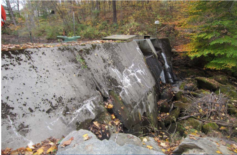
Louis Enten Pond Dam #1, Putnam Valley, NY
